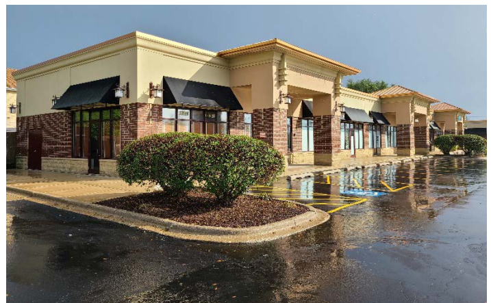
Looking at northwest corner of existing tenant space
